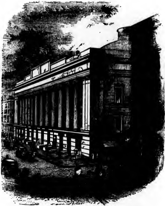
MERCHANTS' EXCHANGE, WALL STREET, NEW YORK.
